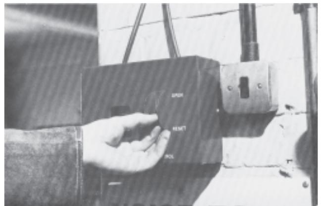
*Fig. 11. Fireman's over-ride control for testing operation of fire vent installation, or for manual operation, when desired*
