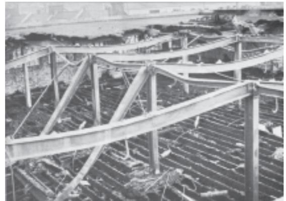
Fig. 04. Steel work affected by fire.
